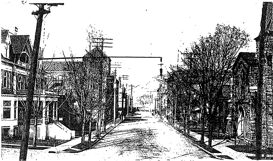
Pine Street Looking North, Corning, N. Y.
