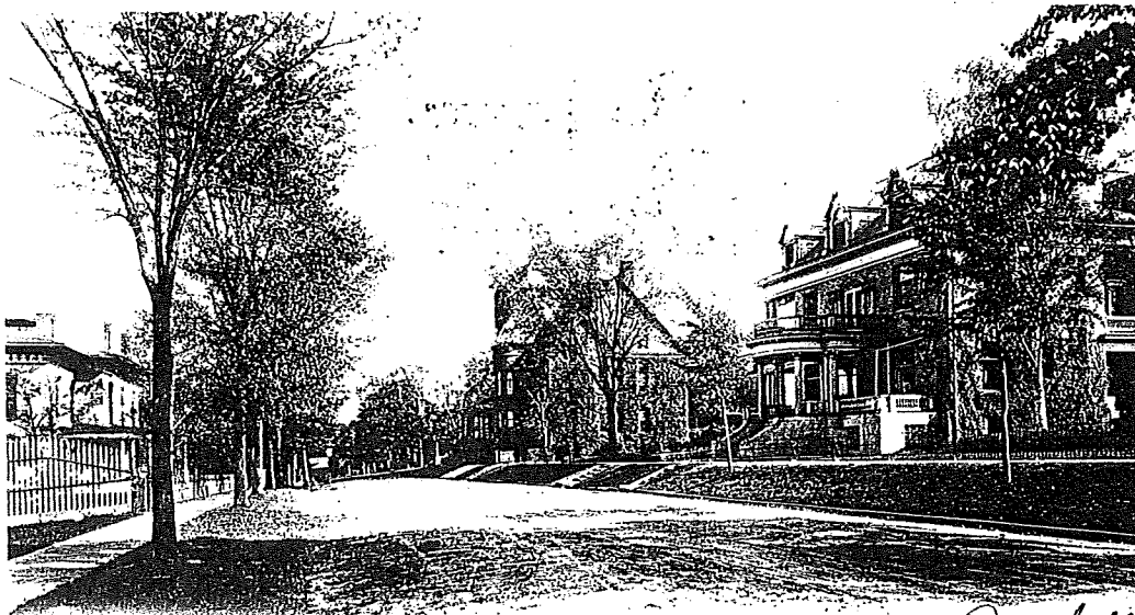
A 25640 Third St. looking East, Corning, N. Y.
